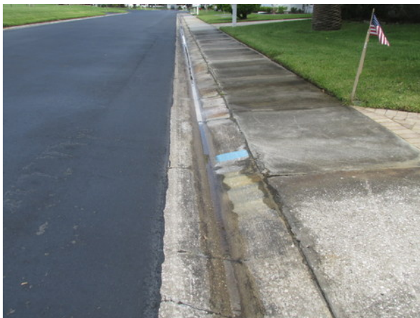
Concrete gutter overview
