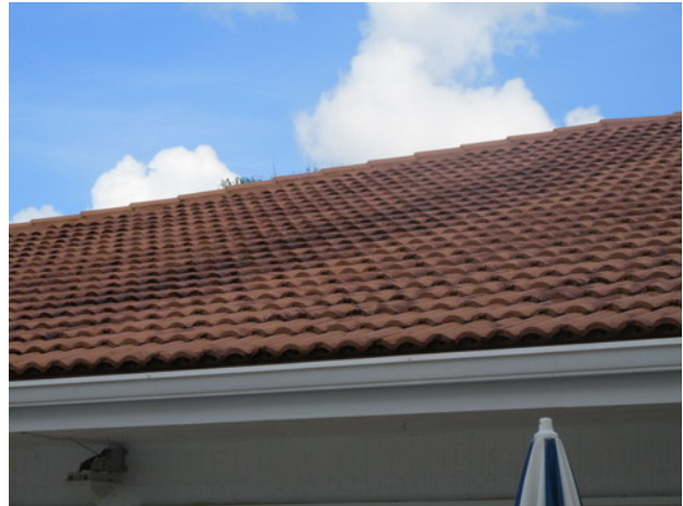
Clubhouse roof overview
