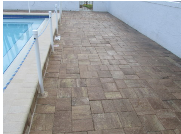
Paver pool deck
