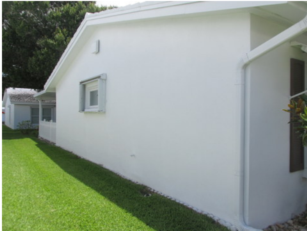
Side elevation overview
