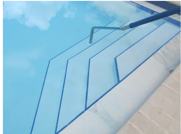
Pool plaster finish
