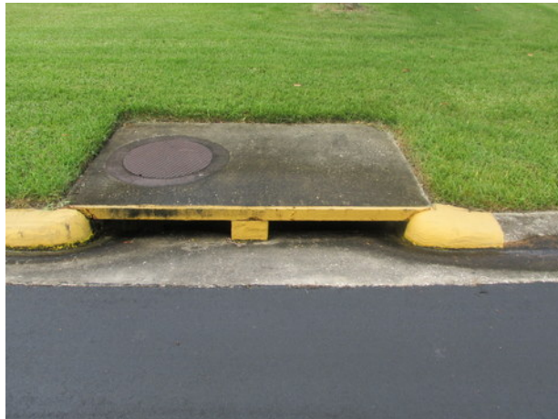
Typical catch basin
