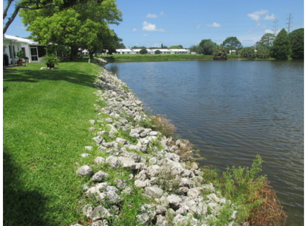
Rip rap shoreline at north pond
