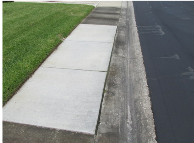
Replaced sidewalk section
