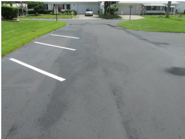
Clubhouse parking area pavement
