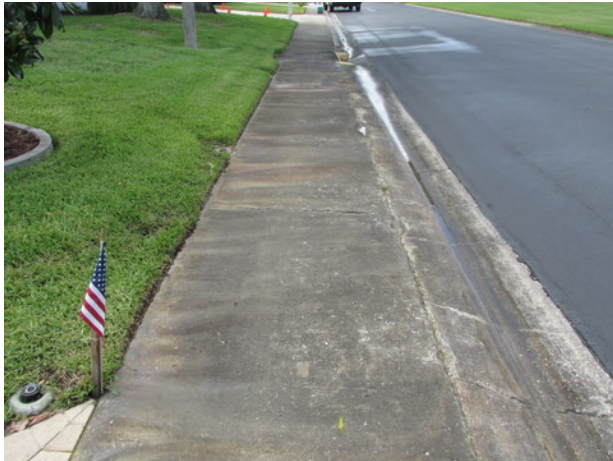
Concrete sidewalk overview
