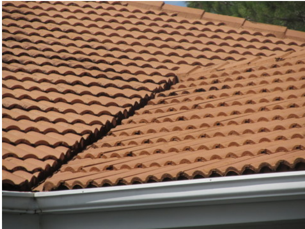
Clubhouse roof overview
