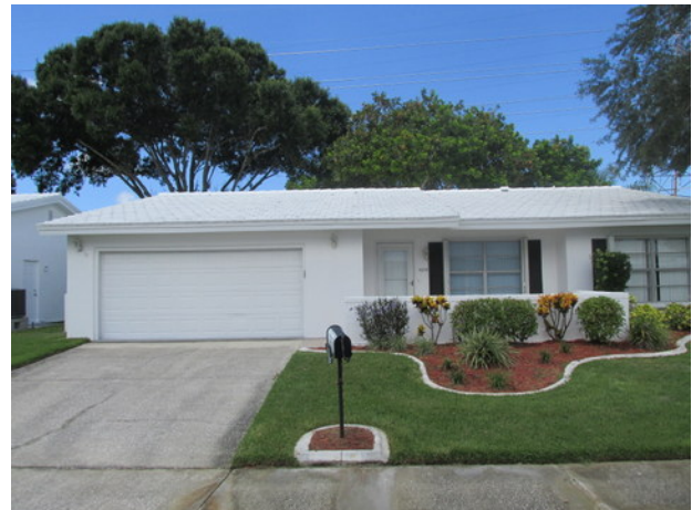
Front elevation overview
