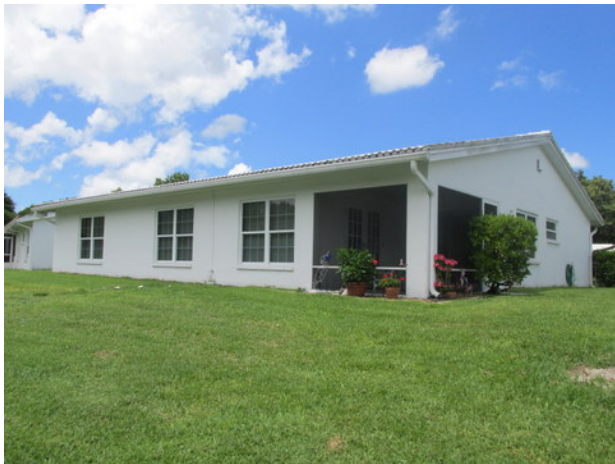
Rear elevation overview
