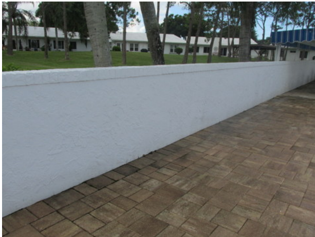
Stucco wall at pool perimeter
