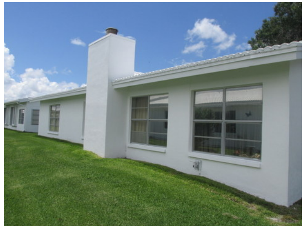
Rear elevation overview
