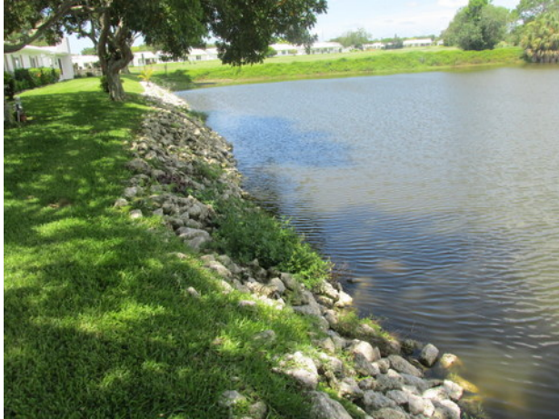
Rip rap shoreline at north pond
