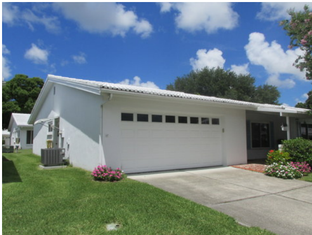
Front elevation overview
