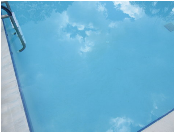
Pool plaster finish
