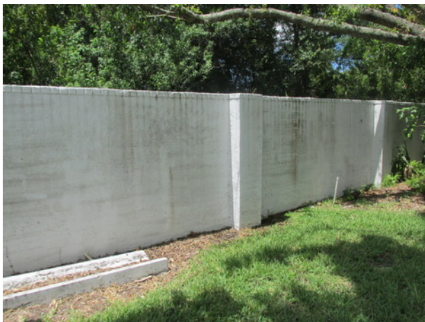
Stucco wall at south perimeter
