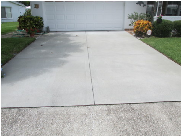
Replaced concrete driveway
