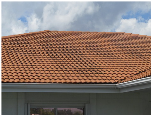
Clubhouse roof overview
