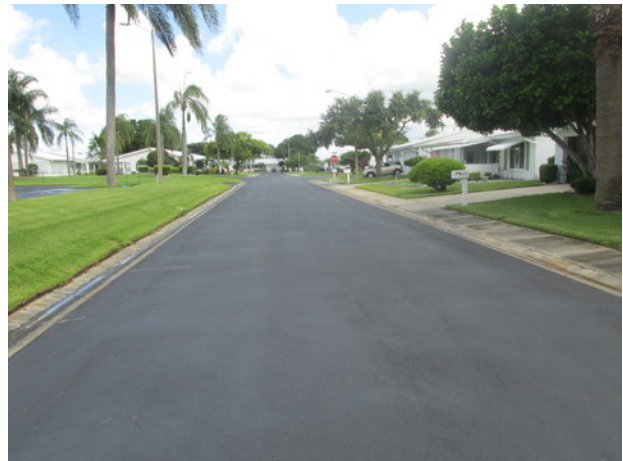
Pavement overview at Mainlands Boulevard
