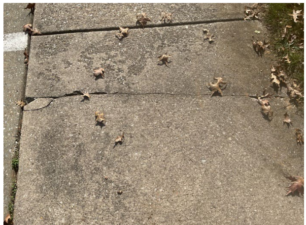
Sidewalk cracks
