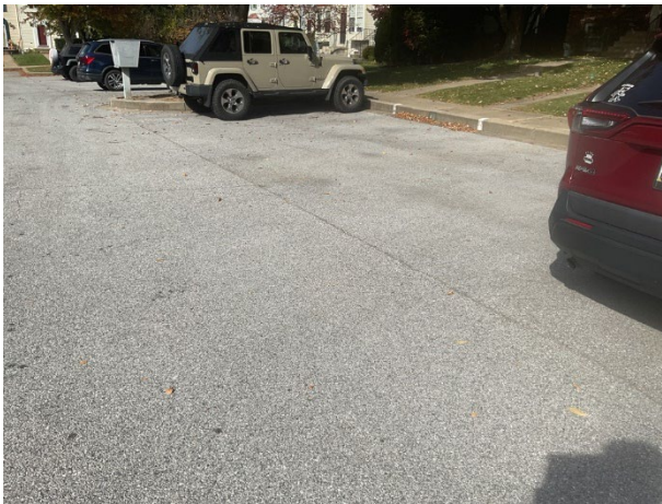
Asphalt pavement parking area
