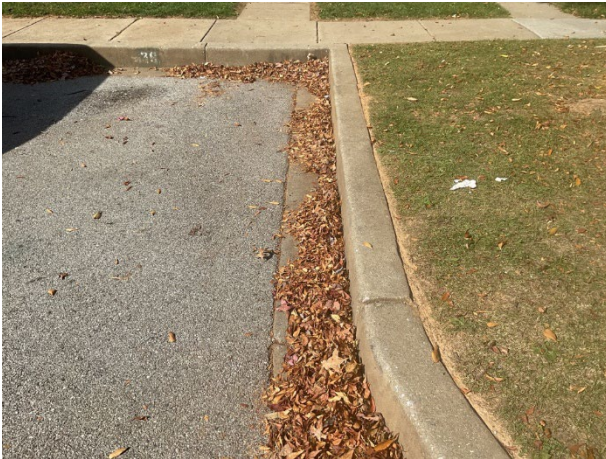
Concrete curb and gutter
