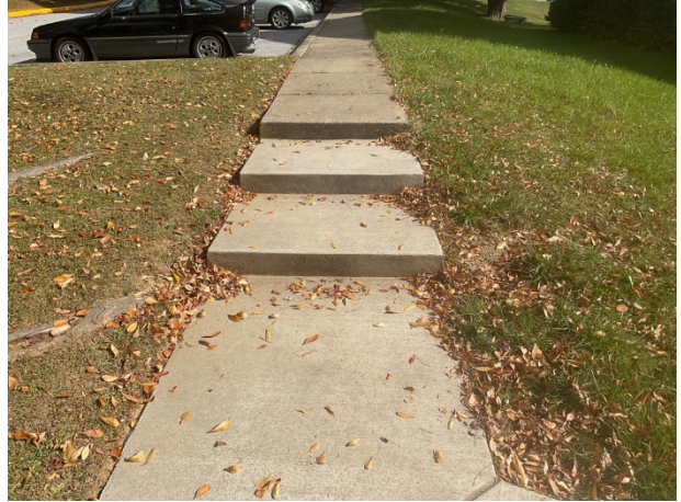
Concrete sidewalk with steps
