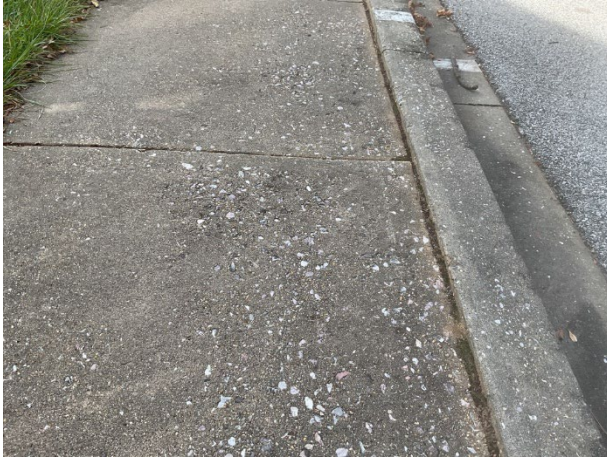
Sidewalk scaling
