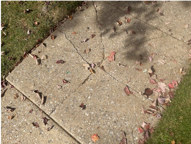
Sidewalk cracks
