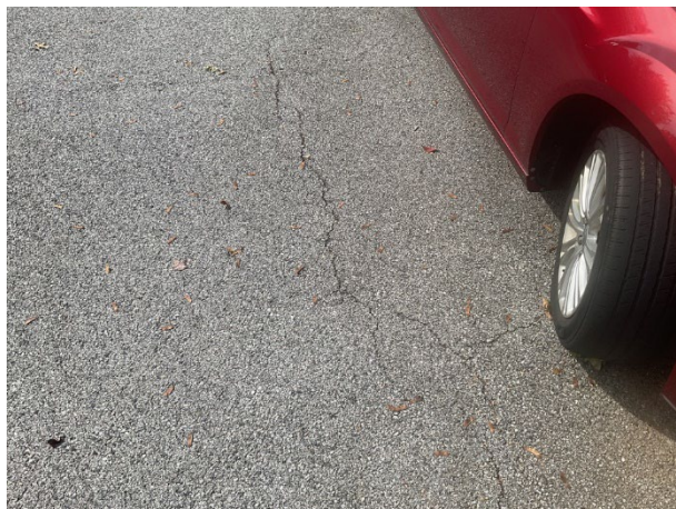
Pavement cracks
