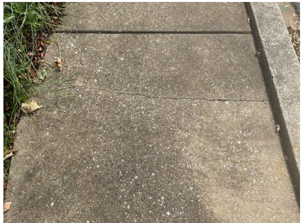
Sidewalk crack
