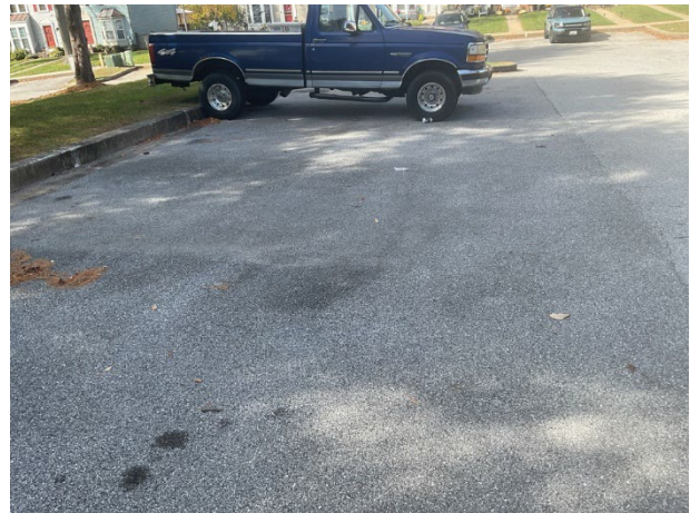
Asphalt pavement parking area
