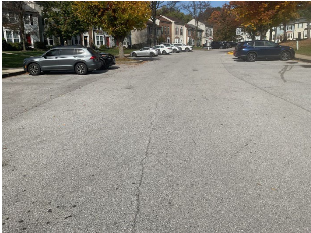
Asphalt pavement street
